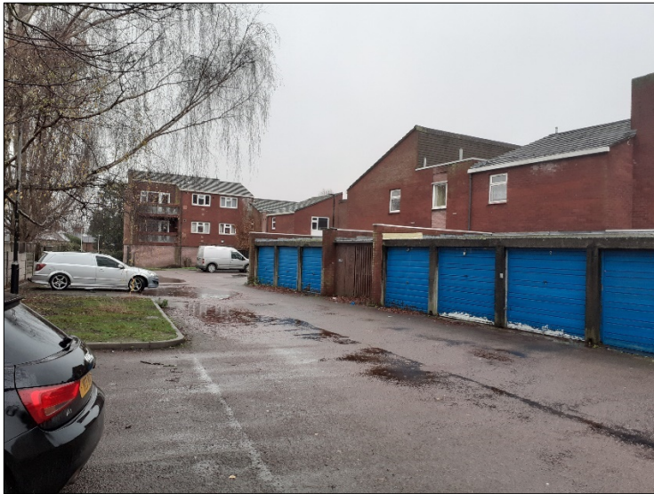
Figure 7 - Garages adjacent to at Fielding Court sheltered accommodation, Loughborough.
